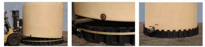
After the stand pieces are tight and the stand is positioned, the molded-in anchor points should be utilized and the tank can be installed following our usage and handling instructions.
