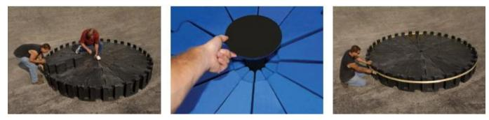
A total of 12 to 18 pieces will be assembled in a circular pattern until the stand is completely assembled. Once assembled, the center pipe and center support plate must be installed. The next step is to wrap a strap around the tank stand and cinch the pieces together. This assures the stand is round by distributing even pressure around the circumference of the stand.
